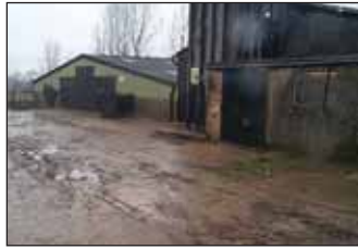
Entrance to Greatwood - before
